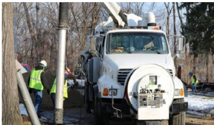
Example of Vacuum Excavation.
